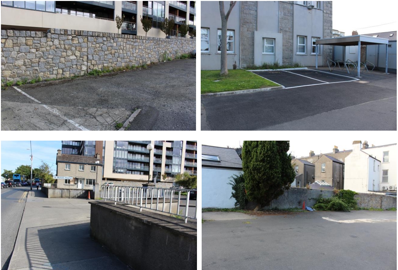
Figure 2 (clockwise from top left): The existing eastern boundary to Harbour View – concrete wall with natural stone on the inside; existing open boundary to St. Michael's Hospital; existing western boundary with various treatments – existing structure, wall with render finish and stone wall with capping; the existing low wall with railing to northern boundary with Crofton Road.
