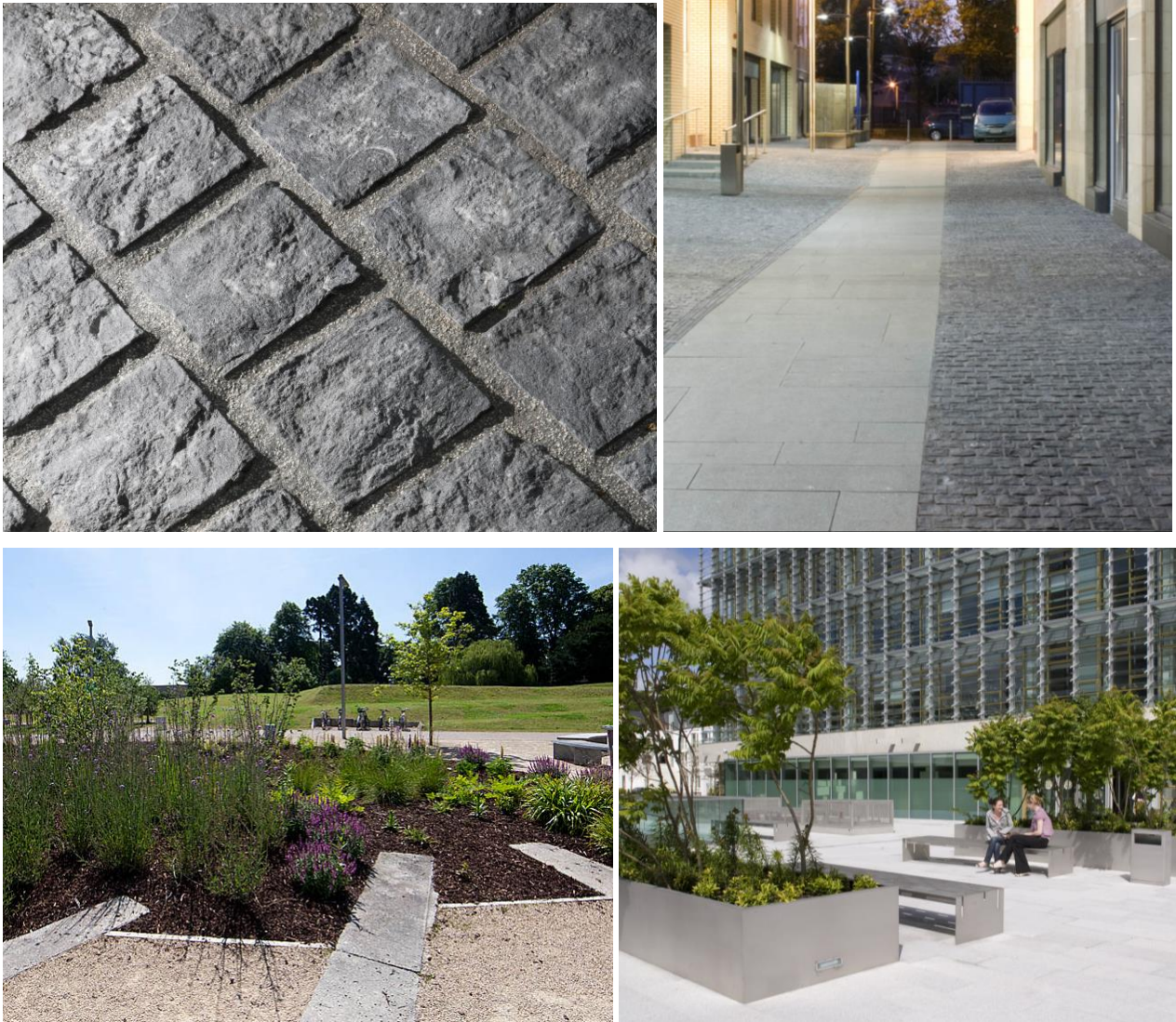
Figure 14: A range of paving details (clockwise from top left): Small format natural stone cubes, streetscape detail with large and small format natural stone paving, raised steel planters and soft landscape sensitively integrated with hard landscape
